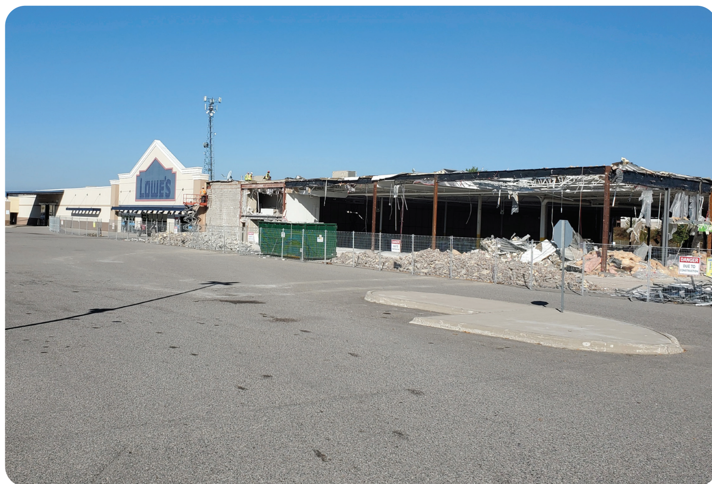
BEFORE Vacant big-box
