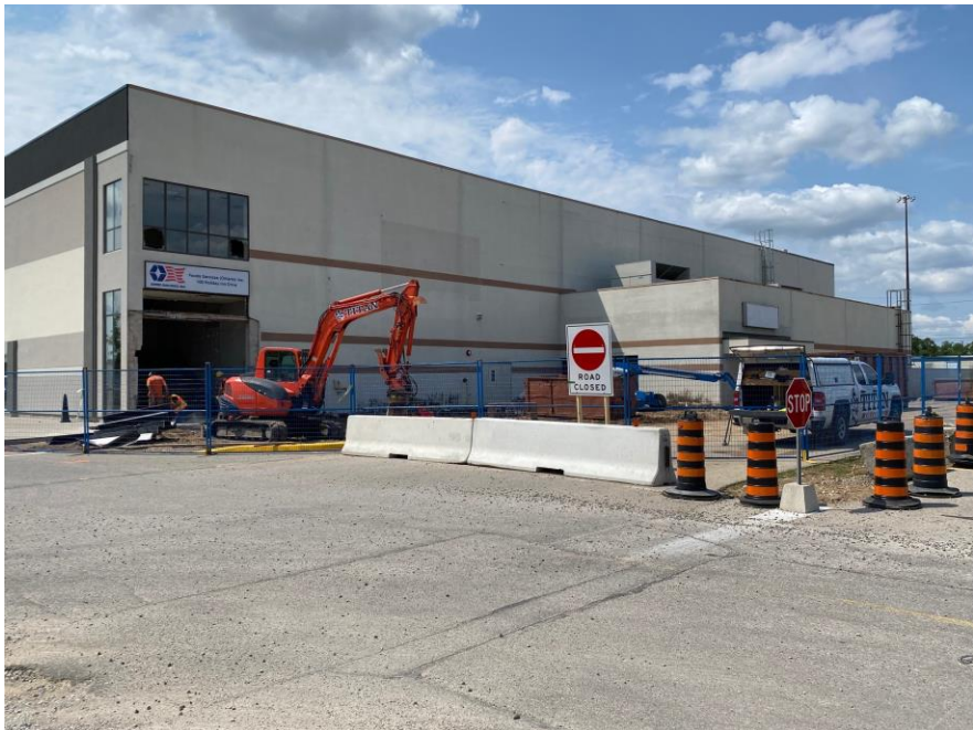
Treasure Hunt - Relocation construction July 2021
